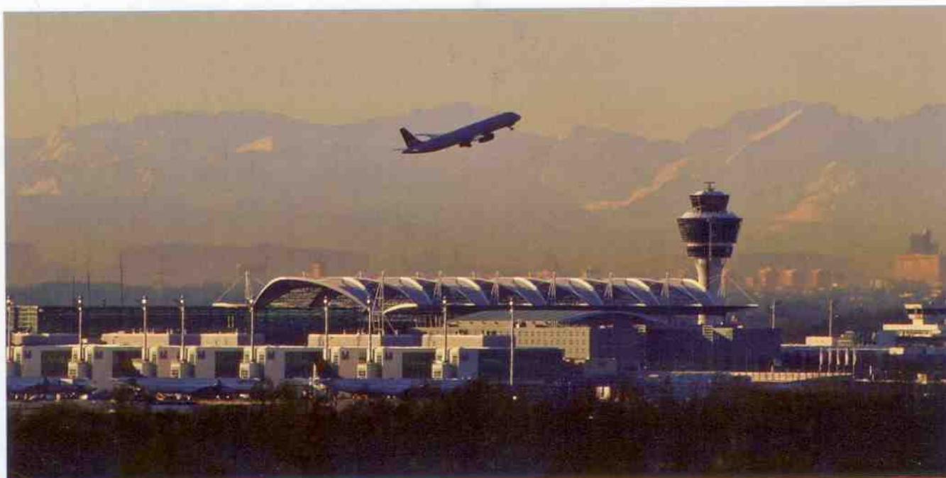
The chief aim of SMS is to detect potential hazards at an early stage
